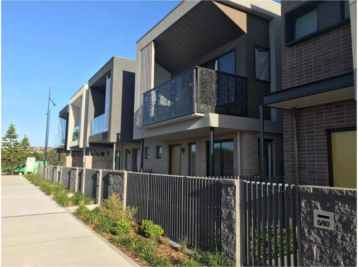
4) Existing dwellings fronting future wetlands area.
