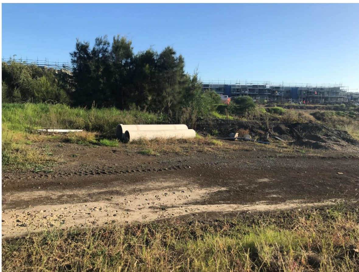
3) View looking north over future wetlands area
