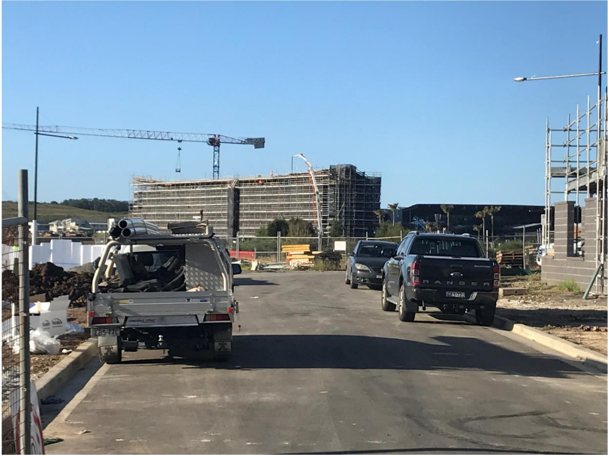
1) View over site looking south towards mixed use development under construction
